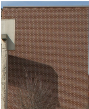
Another wall of bricks
